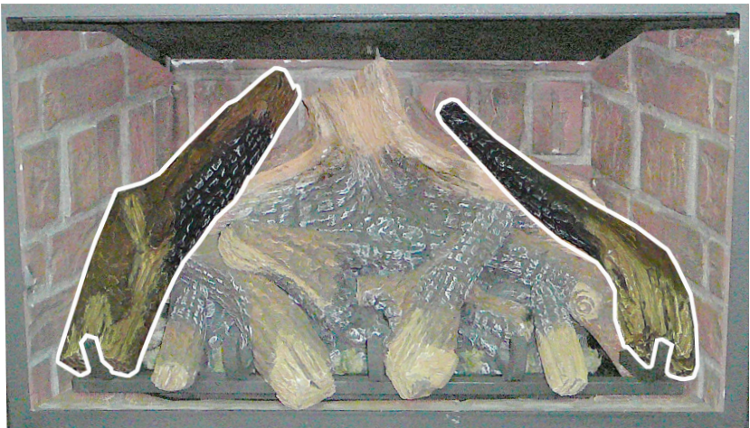
Figure 51. Eighth Stage Log Set Installation.
