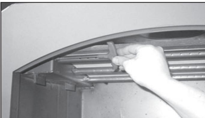
Figure 4.6 Removing Manifold Tube
