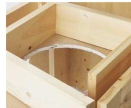
3. To install the ceiling support, just slide the assembly into the framed opening from below. Once you ensure that the finishing plate is flush with the underside of the ceiling and assembly is level, secure it with screws.
