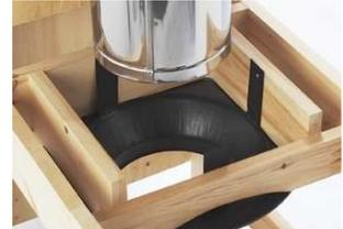
5. Then, from beneath the support, insert the stove pipe adapter and twist-lock it into place.
