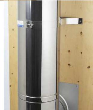
7- Authorities require that the chimney extend not less than 3 feet above the highest point where it passes through the roof of a building and not less than 2 feet above any portion of the building within 10 feet. If the chimney extends more than 5 feet above the roof deck, roof guys with telescoping legs and draw bands are required.
